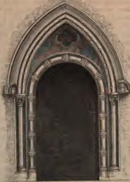
DOORWAY OF THE NORTH TRANSEPT.
